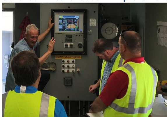
Figure 4- A Brunner Landfill engineering manager discusses the operations and controls of the Heartland Concentrator.
