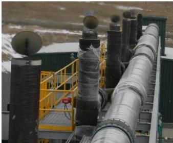
Not only was this a robust mechanical design, but the waste heat provided enough thermal energy to treat the entire produced water stream.
