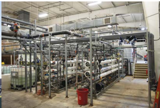
Figure 2: Concentrated leachate from the RO Plant requires treatment.
