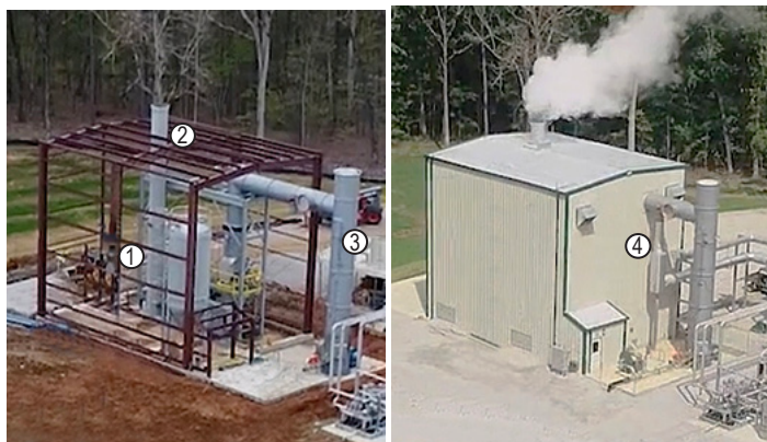
Three Rivers Concentrator during (left) and after (right) construction
